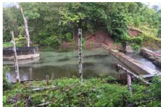
d) Check dam
